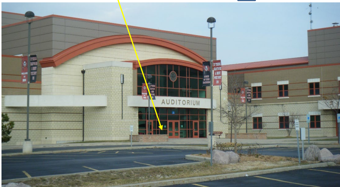
DOOR 4: MAIN AUDITORIUM ENTRANCE
